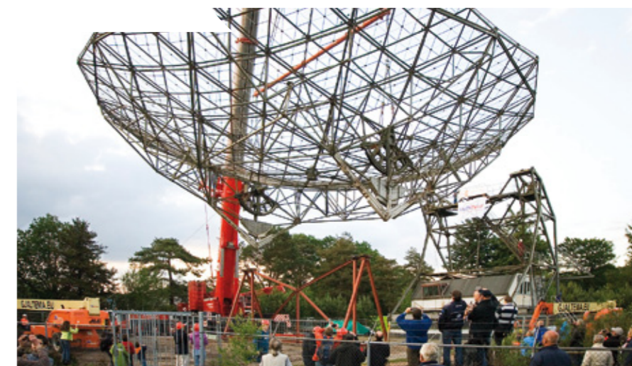
The dish of the Dwingeloo Telescope came off its tower for restoration. The Dwingeloo Radio Telescope was, at the time of its opening in 1956 by Queen Juliana, the largest radio telescope in the world. Until the '90's of the last century, the telescope has served as a scientific instrument. Astronomers mapped our galaxy with the Dwingeloo Radio Telescope. In 1998, the 25-meter dish, was placed in the so-called storm position and since then, has no longer been used for scientific purposes. The Dwingeloo Radio Telescope is a protected monument since 2009 because of its history and (international) scientific significance. With the establishment of the CAMRAS foundation in 2007 ( www.camras.nl ), the radio telescope has been given a new purpose for amateurs and education.
