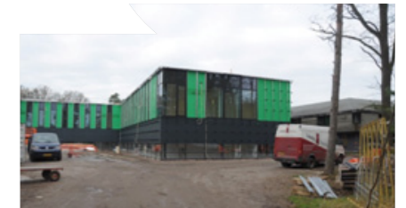
The new wing of the ASTRON building during the building process.
