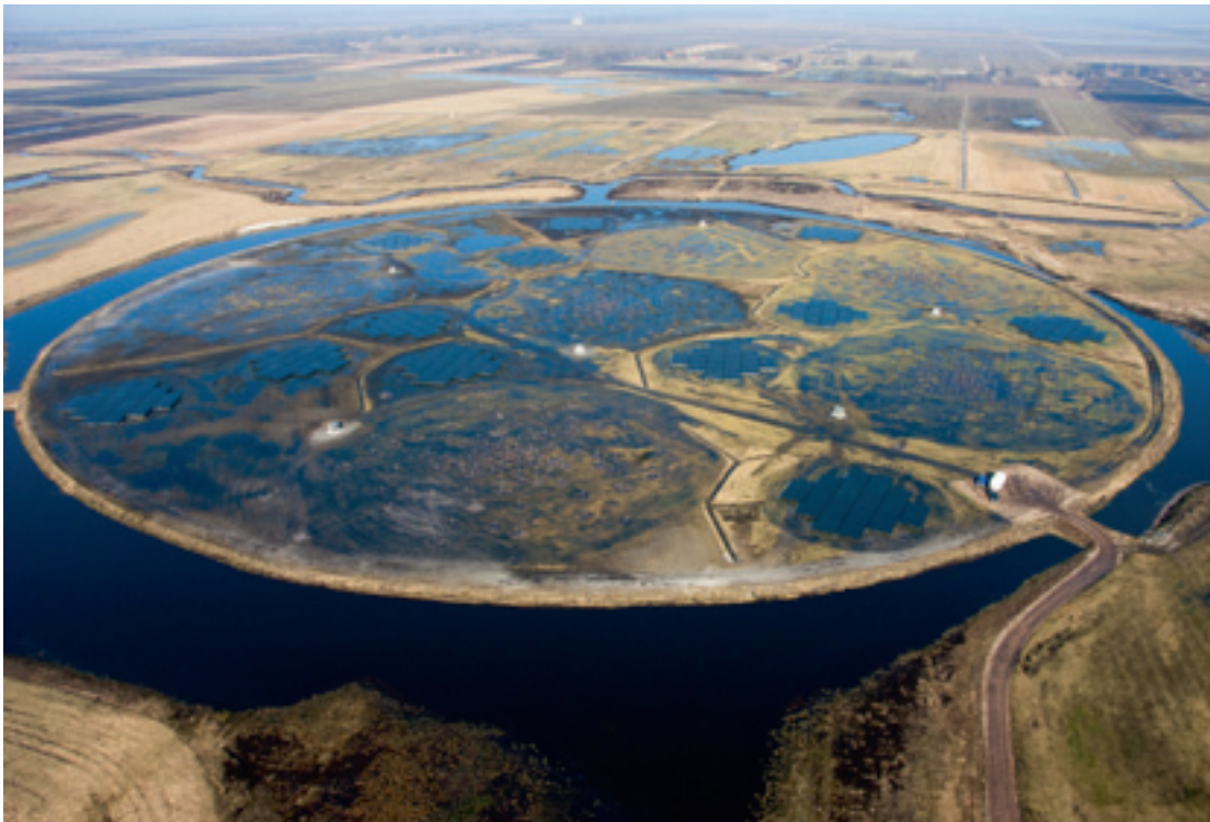
In March 2010 the LOFAR superterp began to emerge from the central core region.
