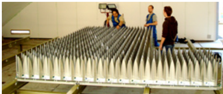
Installation of the null-series tiles in the radome at Westerbork
