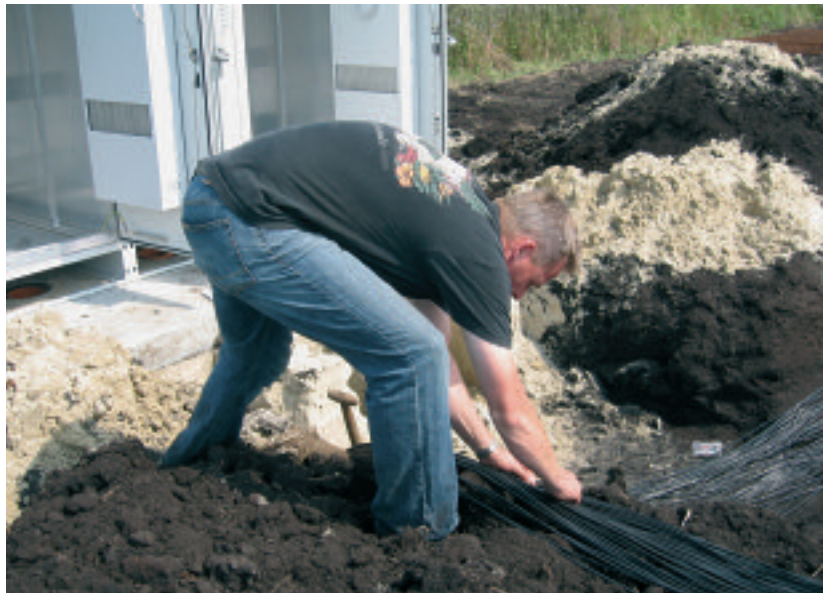
In the second half of 2006, LOFAR Core Station 1 was built. The picture shows LOFAR Roll out manager Mark Bentum, feeding the antenna cables to the electronics cabinet.
