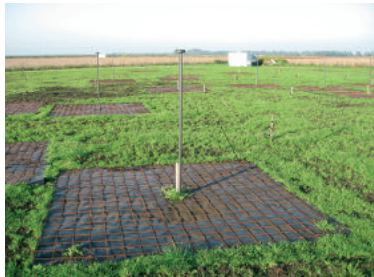
LOFAR low-band antennas at Core Station 1.
