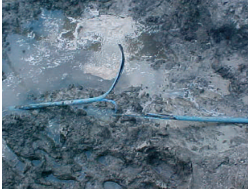
On November 1st 2006, the backbone of LOFAR was broken due to constructions along the A28 highway. All 144 fibers had to be welded on two places to restore the 65 kilometer fiber connection, after which LOFAR CS1 tests could be continued.
